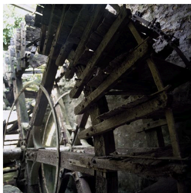
Roue hydraulique verticale. Phot. Olivier Coquelle IVR22_19946000943XA
